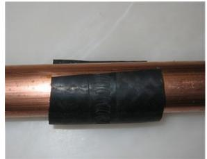
3. Place a Stainless Steel hose clamp over the rubber hose DIRECTLY over where the pinhole is located. Tighten the hose clamp securely. This should force the rubber hose into the pinhole and temporarily stop the leak.
